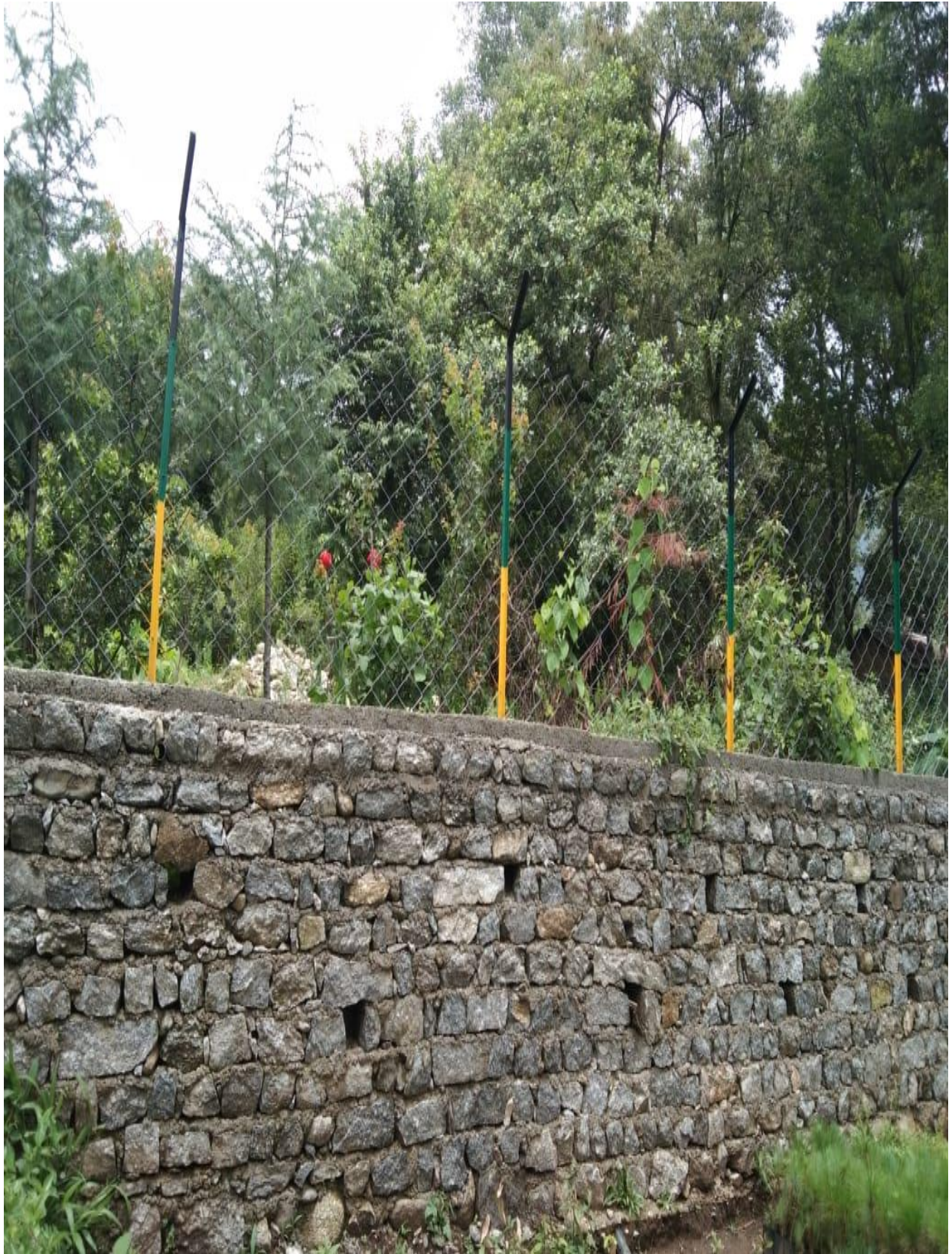
Nurseries Established Under PIHPFEM&L (JICA Assisted Project)
